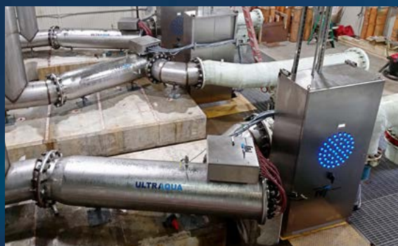
LARGE SCALE AQUACULTURE, USA Large closed reactors for RAS fish farm.
